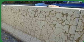
Alkali Silica Reaction (ASR)
